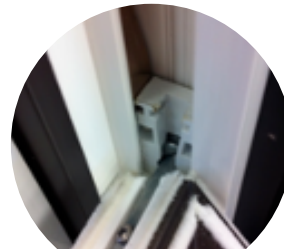
Stainless Steel Constant Force Balance System
